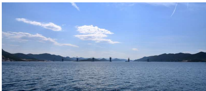
most v gradnji .... work in progress .....
